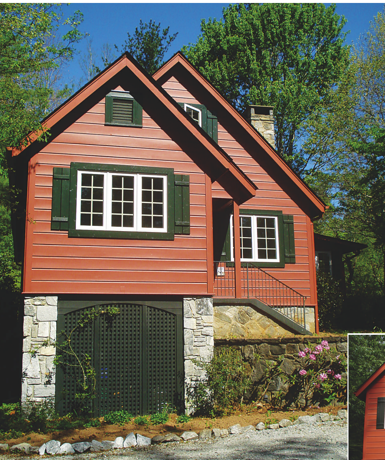
First Restoration of Asheville replaced the odd-size, metal-frame, single-pane windows with vinyl-clad insulated look-alikes in standard sizes. Custom Dutch lap siding fills the gap in the original window openings.
